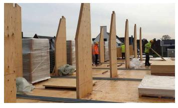
Figure 1. Machined Kerto LVL components
